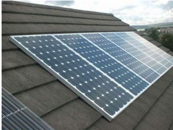
Font: Solar EnergiesUK Figure 2. Solar Panels
